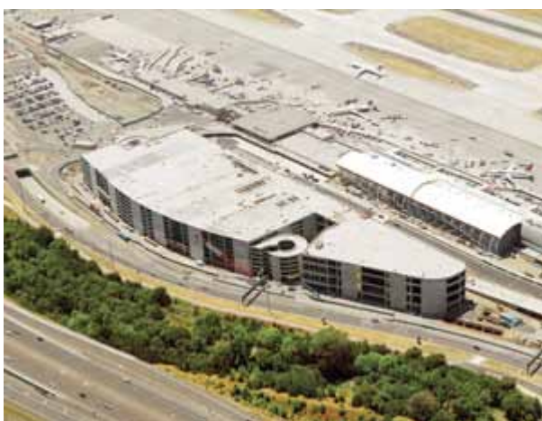
No. 32 Clark Pacific supplied the concrete work on Mineta San Jose Airport's car rental facility.
